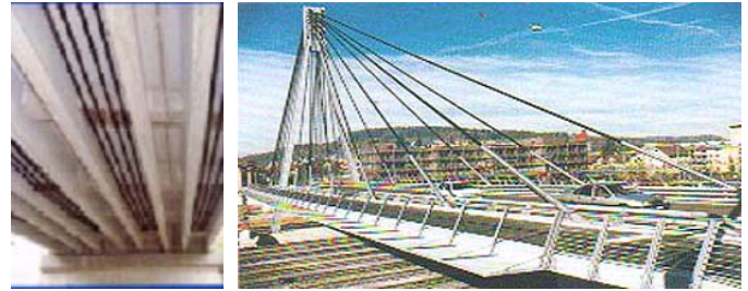
Figure 5 Left Southfield Bridge, Michigan, Right, Storchen Bridge
